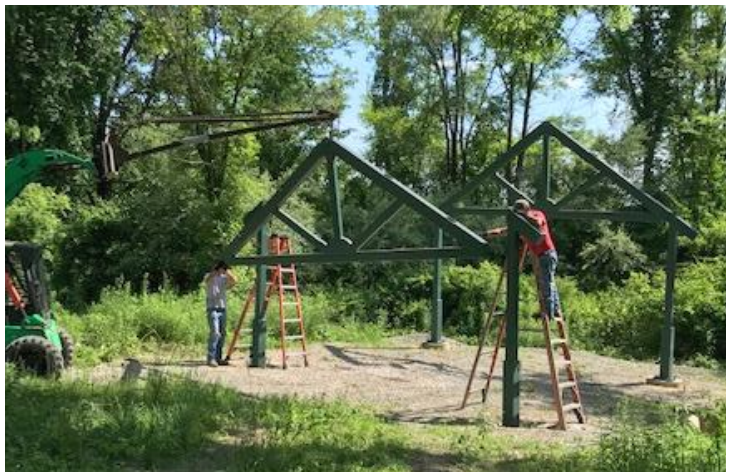
Coverworx employees installing pavilion at Marsh View Park.
