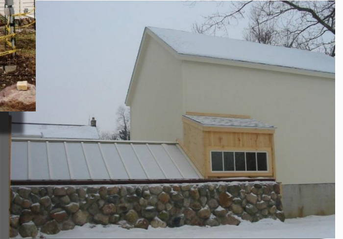
Greenhouse before and after restoration
