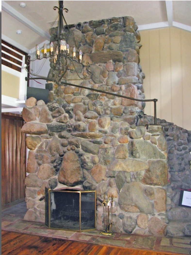
Unique fieldstone fireplace that includes staircase running through the fireplace.
