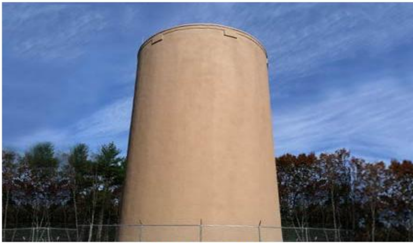
Water Storage Tanks 0.70 MG Water Storage Tank Engineer: Underwood Engineers
