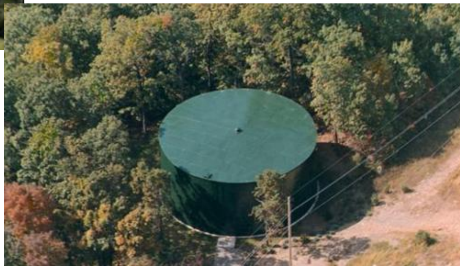
Painted Steel Ground Water Storage Tanks
