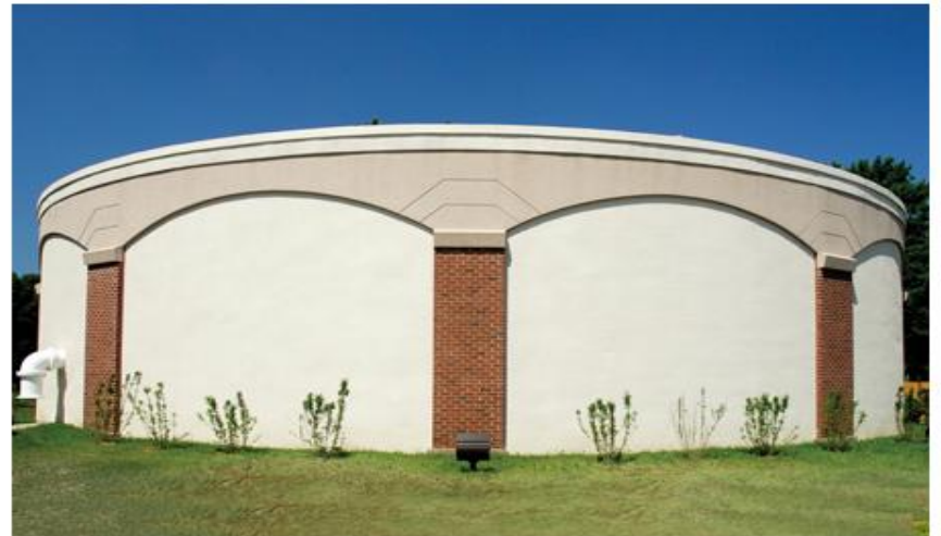
Water Storage Tanks 1.0 MG Ground Storage Reservoir Engineer: Robinson Engineering, Ltd
