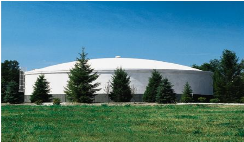
Water Storage Tanks 2.0 MG Water Storage Tank (BW) Engineer: Board of Water & Light, Engineering Dept.
