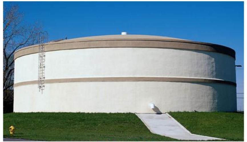
Water Storage Tanks 1.25 MG Water Storage Tank Engineer: Akhras Associates, Inc.
